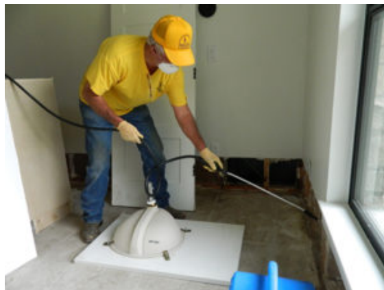
Elvin Bowman, a Texas Baptist Men volunteer from Wylie Baptist Church in Abilene, sprays disinfectant, providing mold mediation for a water-damaged home in Granite Shoals. (Photo / Ken Camp)
