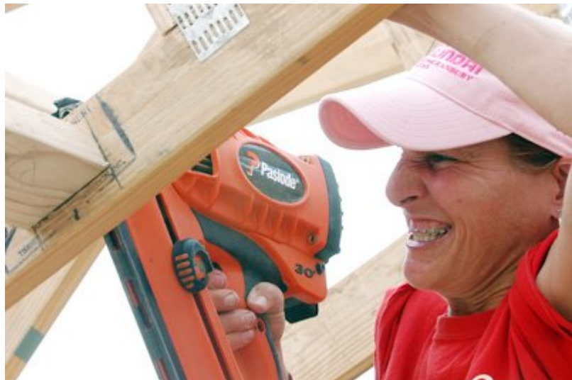
Shelly McQuarie from First Baptist Church in Cleburne uses a nail gun in installing trusses for the roof. (PHOTO/John Hall/BGCT)
